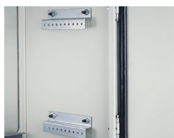
Perforated rails installed on lateral studs.
