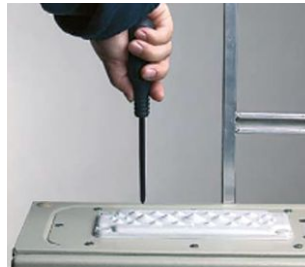
Make a small hole in the membrane.
