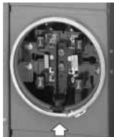
Manual Slider-Type Bypass Shown in Open Position with Handle Secured by Notch Meter Socket Sealing Ring
