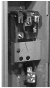
225 A Q-Frame Tenant Circuit Breaker Base (Three-Pole)
