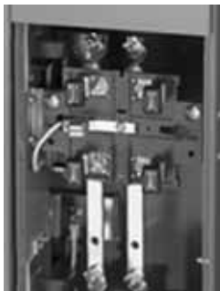
Five-Jaw Kit (5J) Installed at the 9 O'Clock Position
