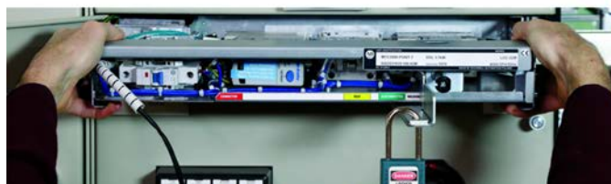
Withdraw lever in the Released position (and locked out).
