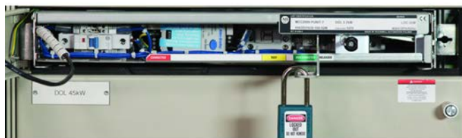
Withdraw lever in the Disconnected position (and locked out).
