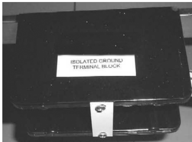
Figure 2.41 Isolated Ground Terminal Block (110...1200 A)
