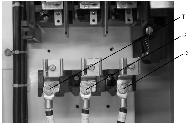
Figure 3.4 Load-side of Circuit Breaker
