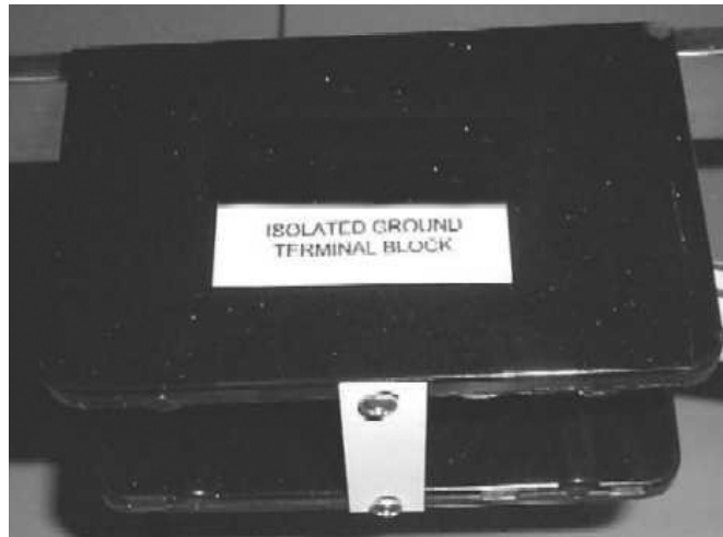
Figure 5.18 Isolated Ground Terminal Block (110...1200 A)
