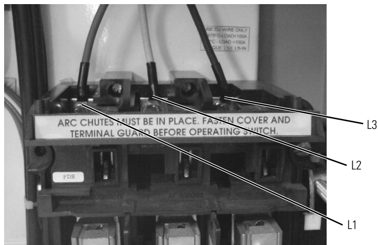
Figure 2.43 Incoming Power Connections on Fusible Disconnect Switch (Bulletin 2032)
