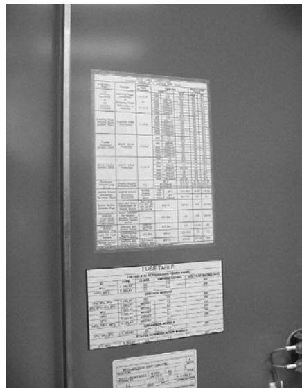
Figure 3.7 Torque Label Location
