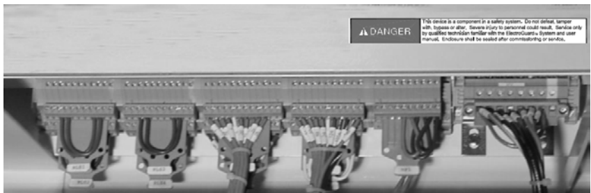
Figure 3.9 Remote Lockout Stations Connector Plugs
