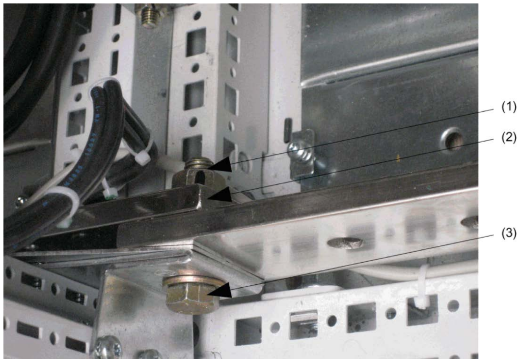
Figure 4-3 Connecting the PE busbars
