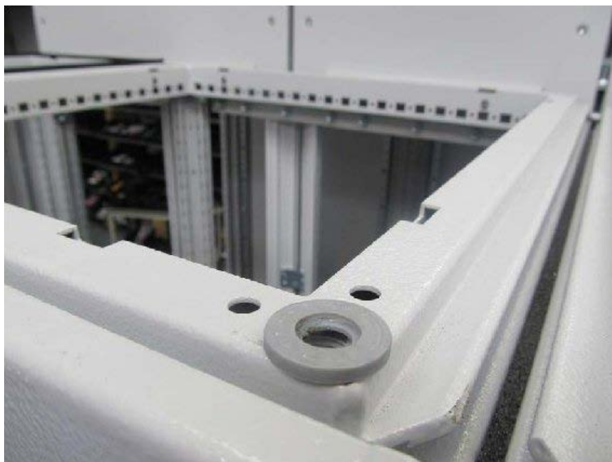
Figure 3-18 Attaching the washers
