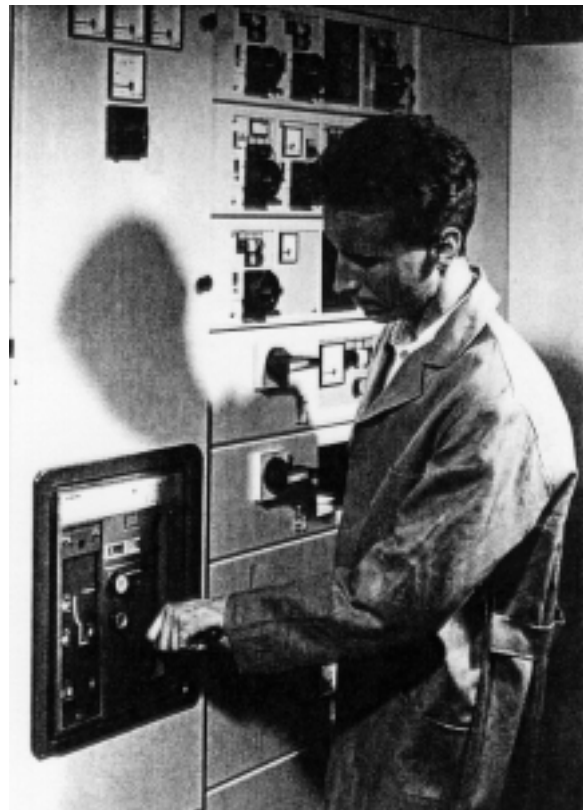
Fig. 1/1 3WN6 in a switchgear installation
