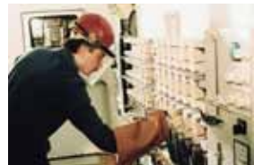
Fig. 3.2.4 – Actuating LV HRC fuse links under load
