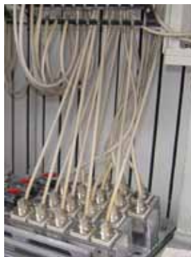
Fig. 3.8.2 – Sand filling for LV HRC fuse links
