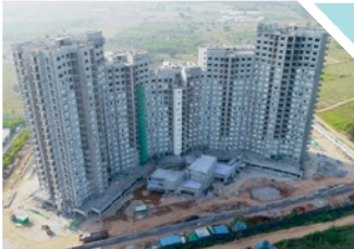
High-rise residential project, Bangalore
