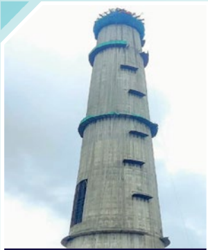
Flue Gas Desulfurisation project, Jharkhand
