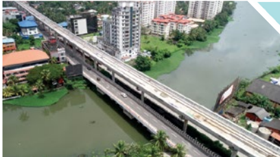
Kochi Metro Viaduct and Panamkuttu Road Over Bridge, Kochi
