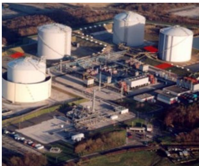
Figure 9: Onshore case study - Decommissioning of a LNG Plant
