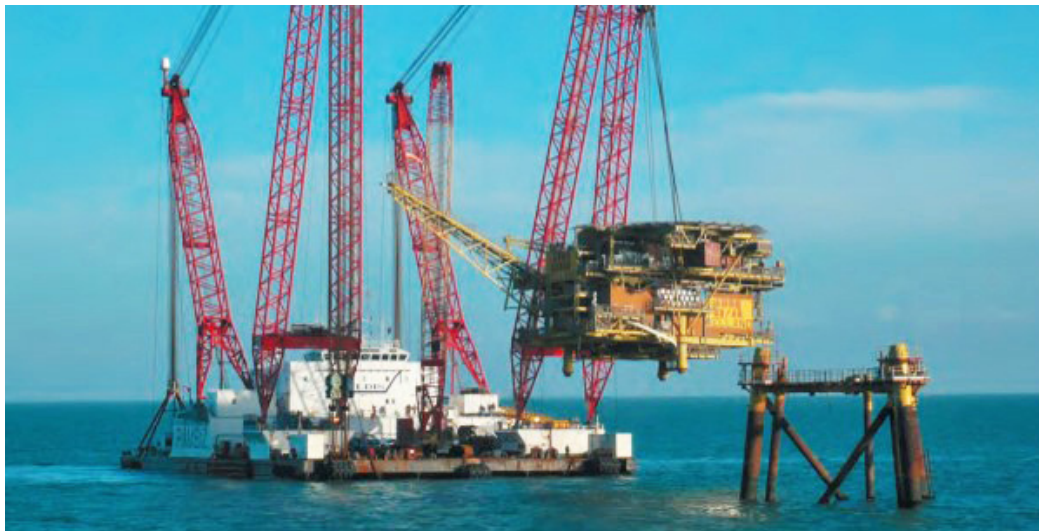
Figure 10: Topsides being lifted off the Welland platform prior to being refurbished and redeployed on a new development in West Africa.
