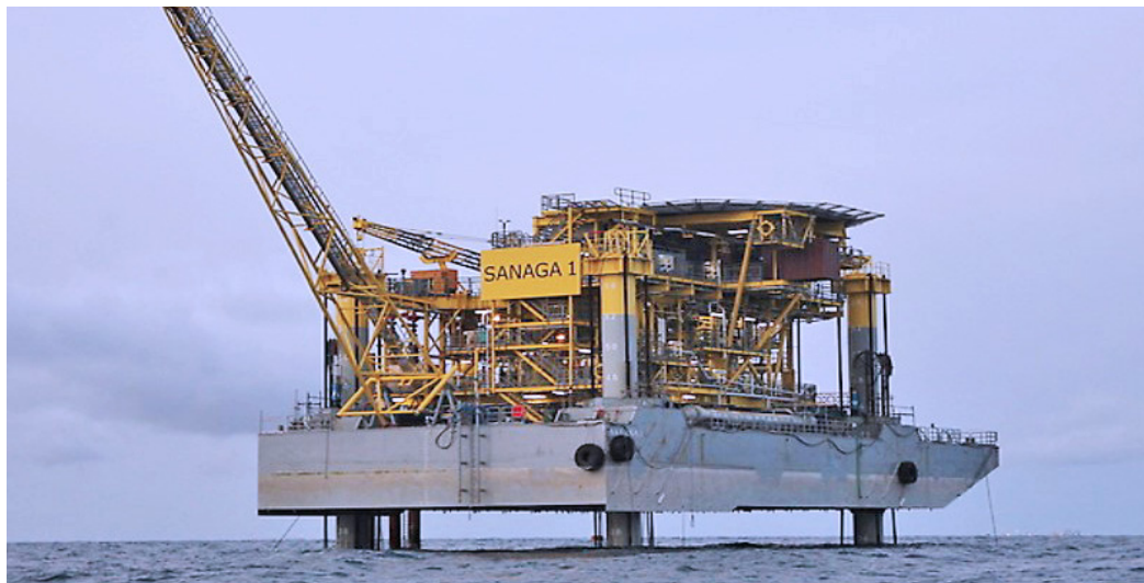
Figure 11: Welland topsides re-used on a new MOPU in the Sanaga field. (Photo from Overdick GmbH.com)
