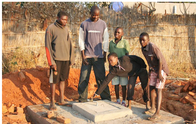
Figure 18: Installation of solar-powered mechanical pump in Africa
