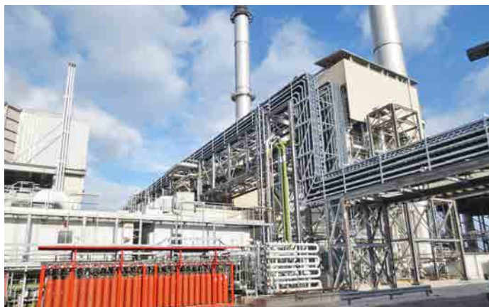
Figure 17: Shotton Power Station
