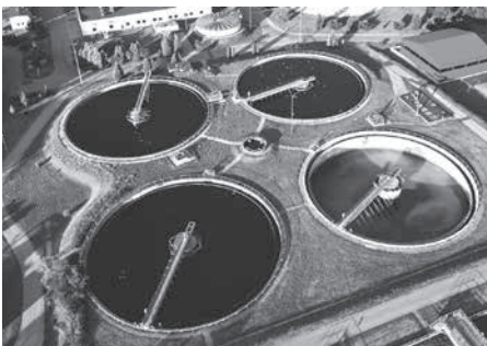
Water treatment system
