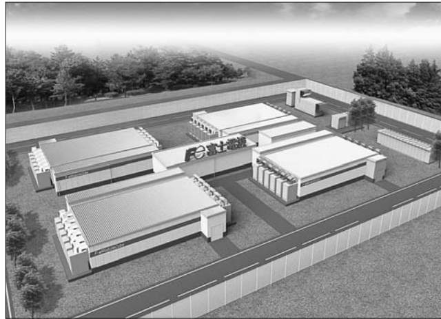
Fig.12 Bird's-eye view of data center site
